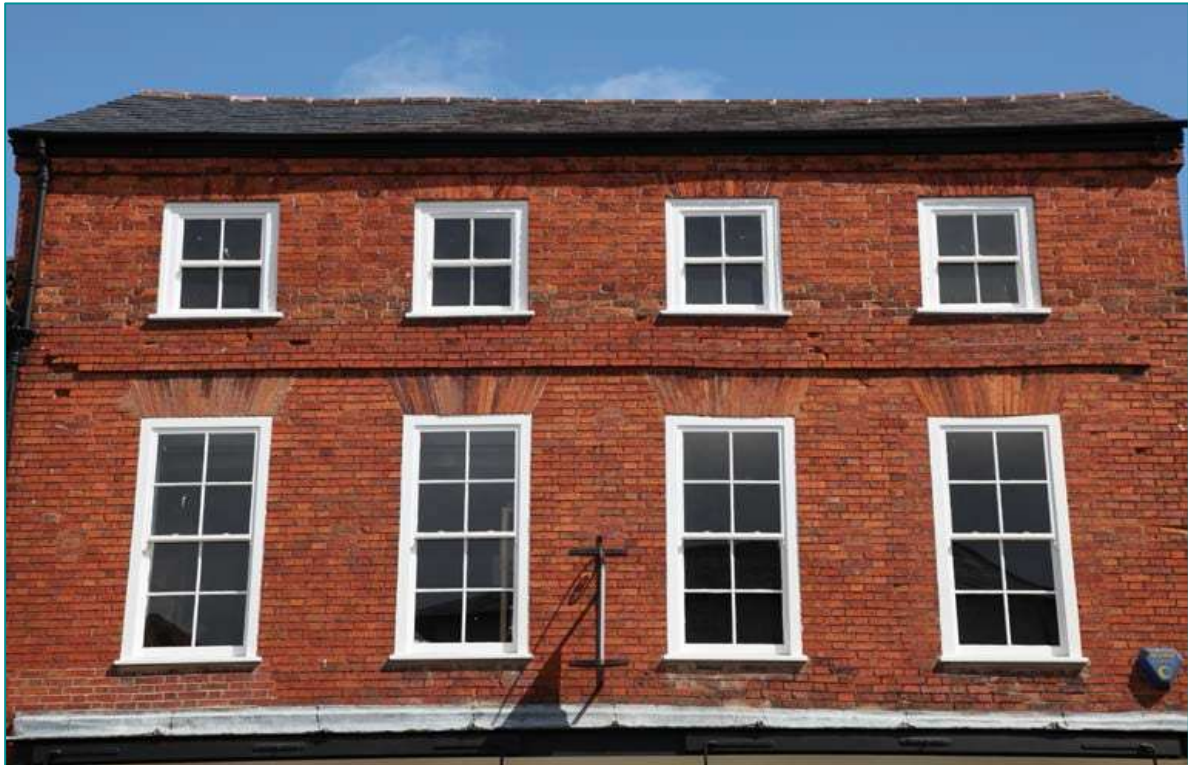
Fig. E9- Gauged brick flat arches on a house in Henley-in-Arden, Arden area. The openings are vertically aligned and the second floor windows are smaller than the first floor windows.
