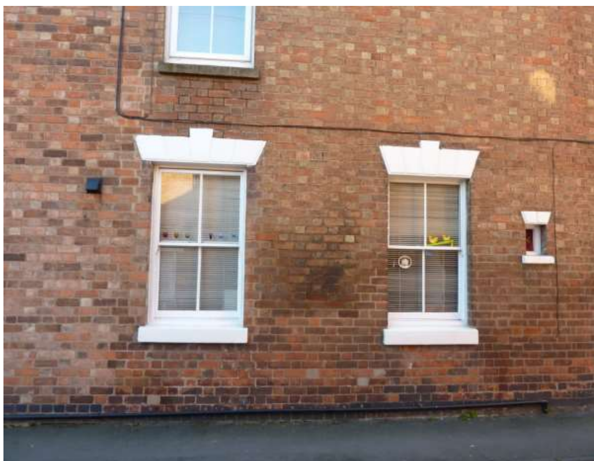
Fig. E12 – An example of windows with render used to create the effect of stone lintels. The windows have stone cills and sliding sash frames.
