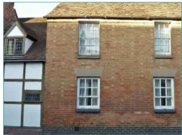
Fig. E2 - Photo of a brick house with rubbed brick flat arch window heads in Stratford on Avon.
