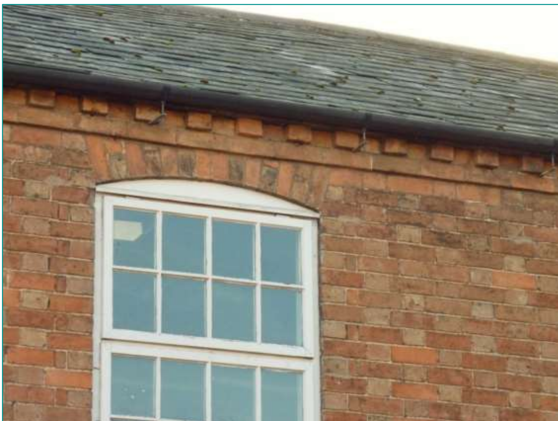
Fig. E16 - Dentilated brick eaves made up of a projecting stretcher course, alternating projecting headers and a further projecting stretcher course.
