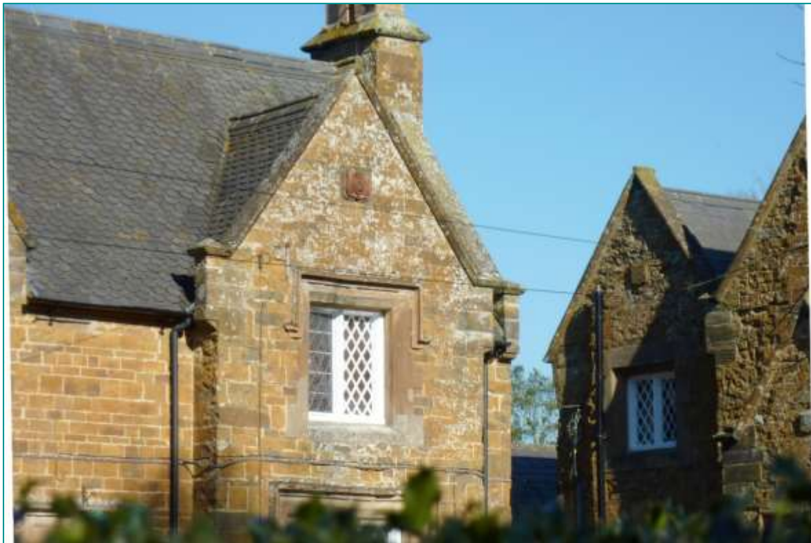
Fig. E15 - A stone-coped gable parapet of Hornton stone with a corbelled verge/eaves junction known as a kneeler.
