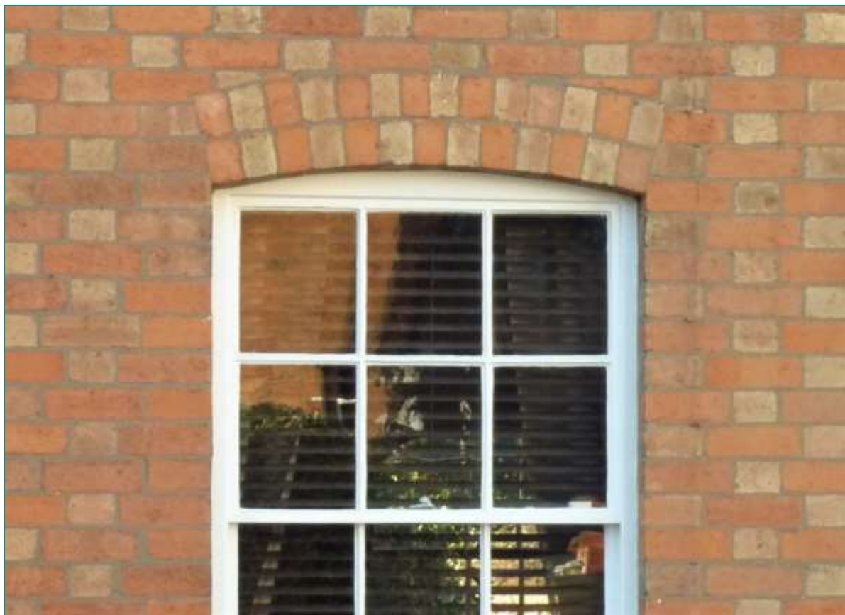
Fig. E10 - Window with a segmental arch head. Note the arch is made up of headers on edge, a detail very characteristic of brick areas within the District.
