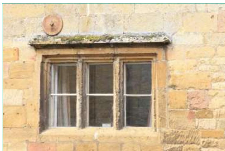
Fig. E13 - A Hornton stone farmhouse with a three light window, stone mullioned window. The window has flush head, jambs and cill with a label or hood mould above the head.
