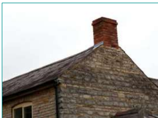
Fig. E14 - Examples of 'wet verge' using mortar to secure the roof tiles.
