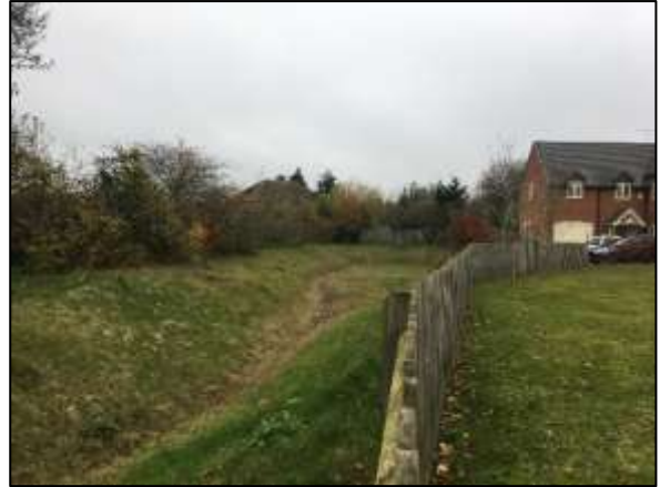
The swale leading to the infiltration basin at Hereburgh Way, Harbury
