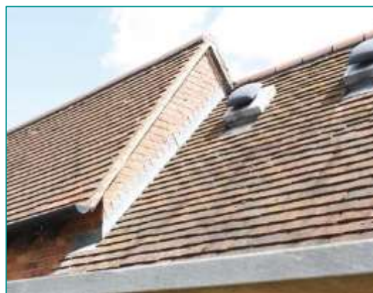
Fig. E14 - Examples of 'wet verge' using mortar to secure the roof tiles.
