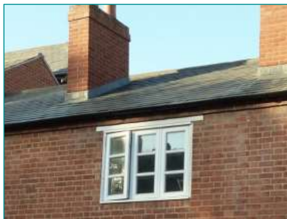
Fig. E11 - Cottages with windows set just below the top plate in Old Town, Stratford-upon-Avon. The casement windows shown are flush closing as opposed to 'storm proof'.
