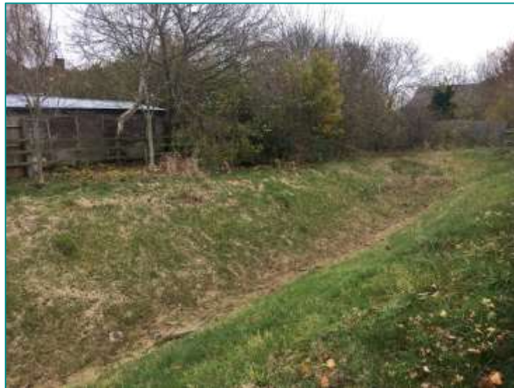
Example of a grass swale in a Harbury housing development. Swales are a type of SuDS consisting of a wide, shallow grass covered depression, leading surface water from a drained surface to a storage or discharge system.
