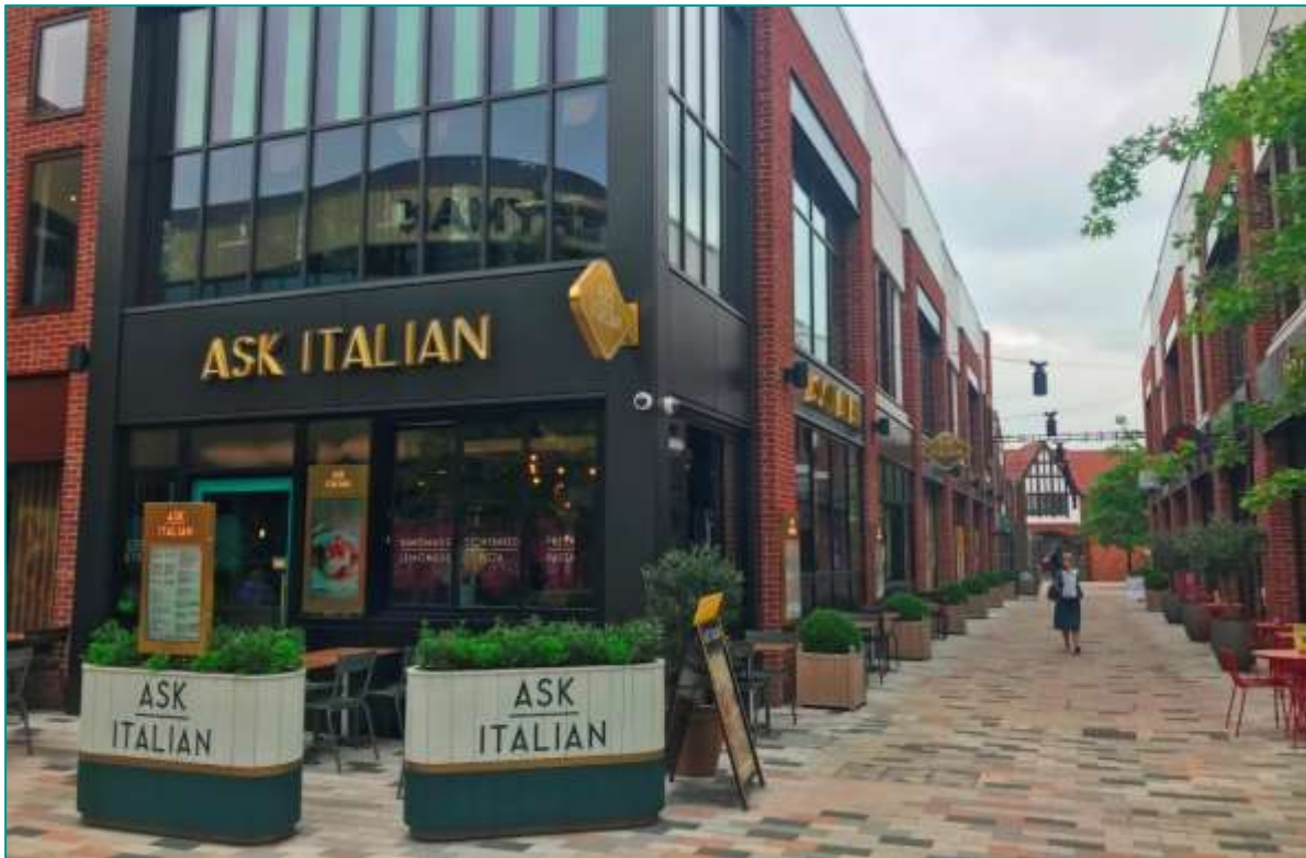
Fig H2. shows a well-designed modern shopfront.
