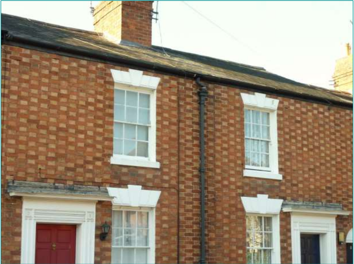
Fig. E6 - Brick (with Flemish Bond pattern using buff brick for the 'header' and orange for the 'stretcher')
