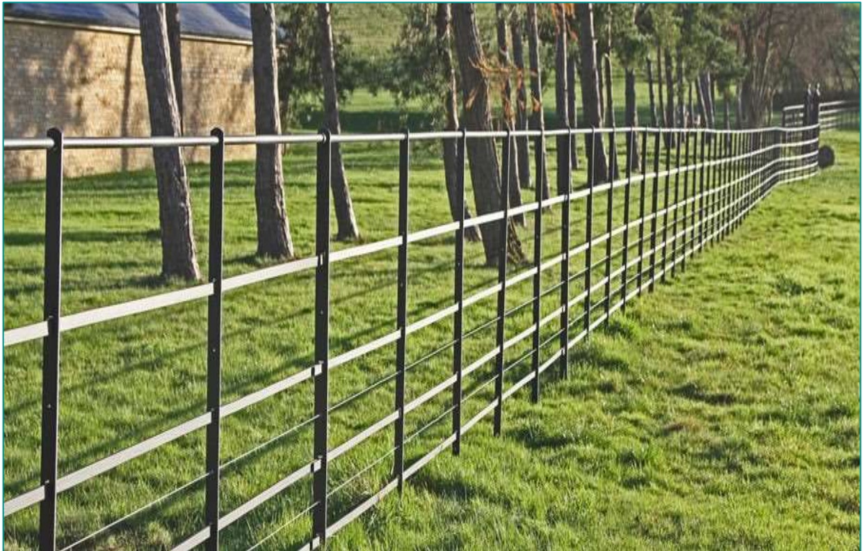
Fig. D12 - An example of estate railings.
