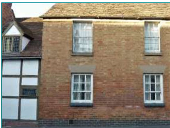
Fig. E11 - Cottages with windows set just below the top plate in Old Town, Stratford-upon-Avon. The casement windows shown are flush closing as opposed to 'storm proof'.
