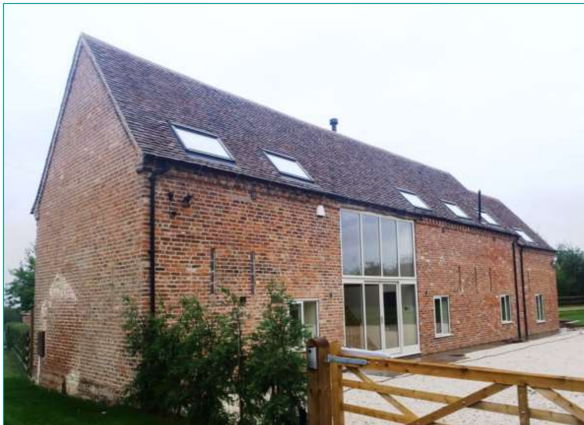
Fig. G6 – An example of well-designed converted barn.
