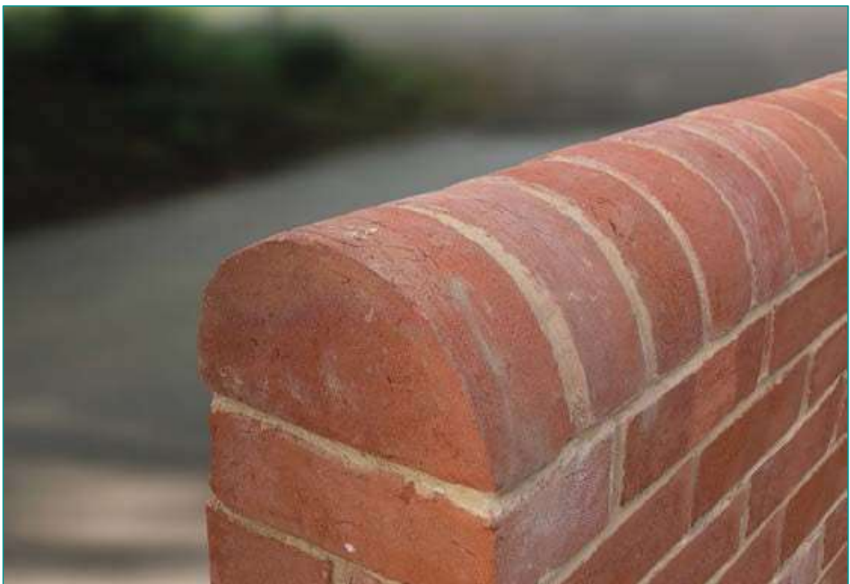
Fig. D11 - An example of a half round copings wall.
