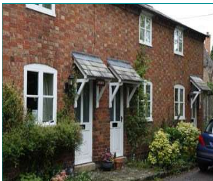
Fig. E22- Lean to canopies with brackets, Welford-on-Avon, Avon Valley. The roof material is inappropriate in this case as smaller roof tiles are needed.
