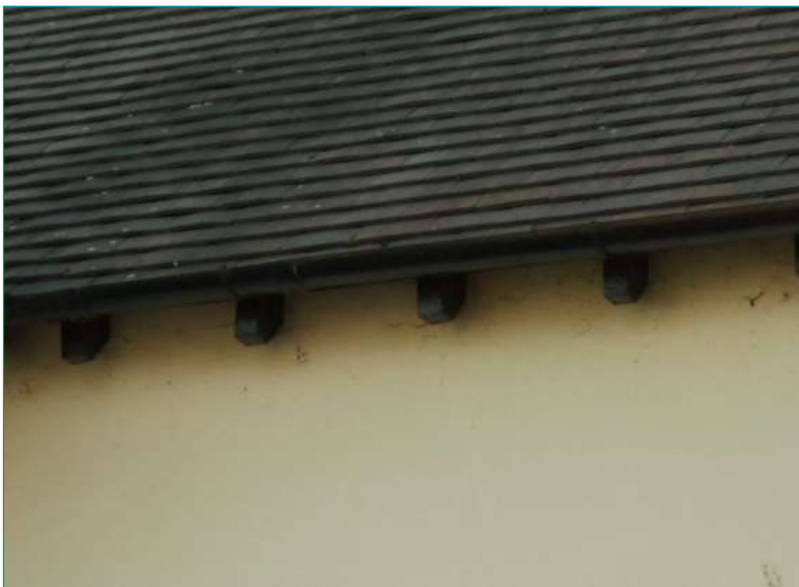
Fig. E18 – Plain eaves with exposed rafter feet on a brick building.
