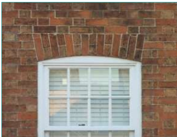
Fig. E2 - Photo of a brick house with rubbed brick flat arch window heads in Stratford on Avon.
